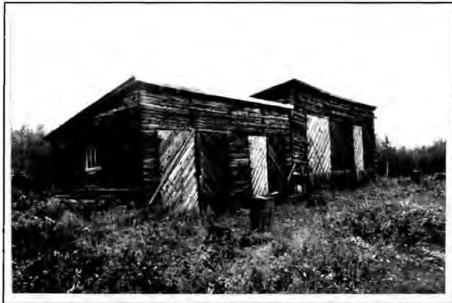
Figure 72. The Turner/Hatten/Agoff Catsheds, 1993. The view is looking northeast.
